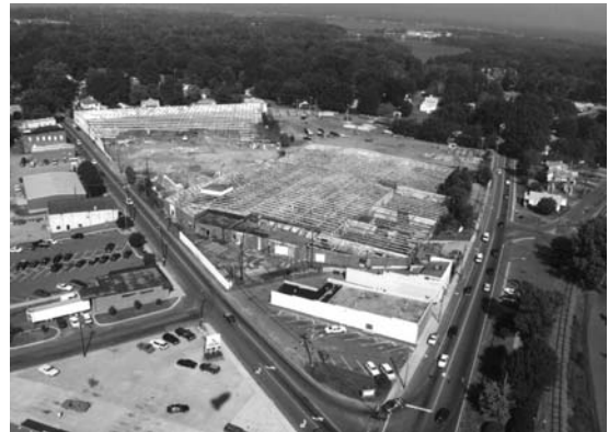
Figure 11.1 Aerial Photo of Cornelius Old Mill Site. This photo from 1997 records the early stages of demolishing the old mill buildings, ugly sheds of no architectural quality. (Photograph courtesy of Shook Kelley architects)
